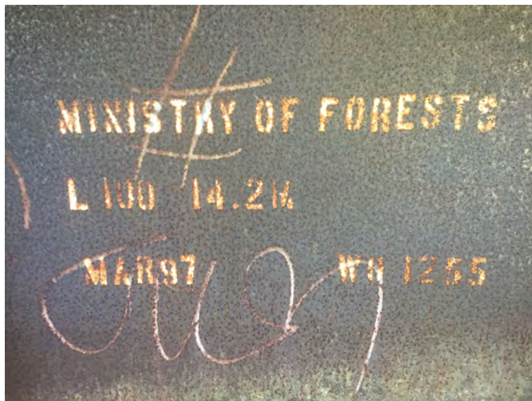
Right span structure ID
