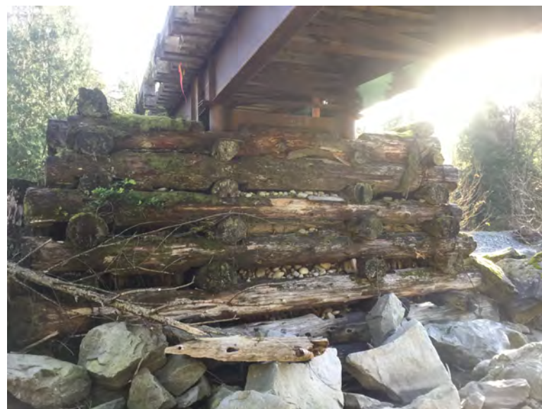
Right face of Pier
