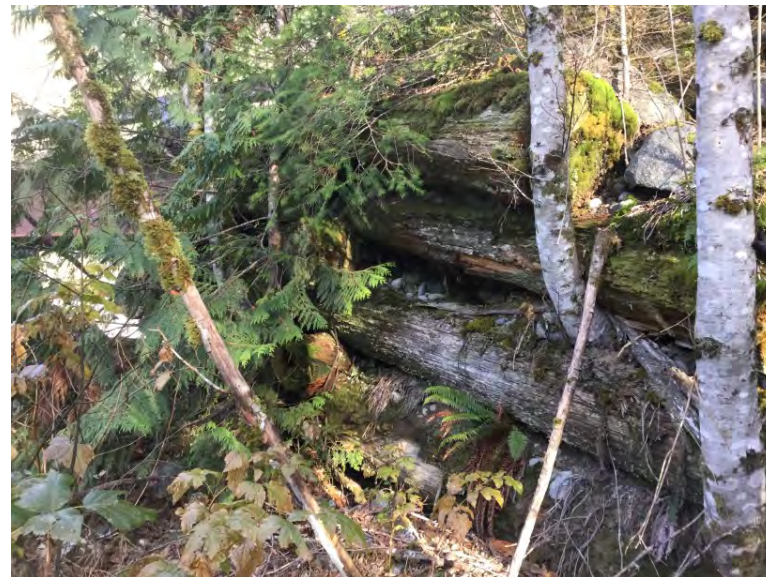
Downstream left bank wingwall condition
