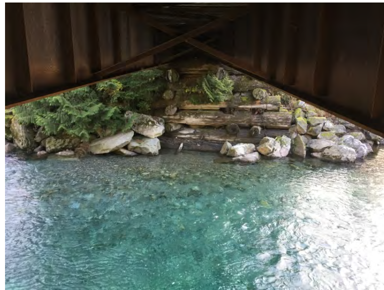
Left Bank Abutment when facing downstream
