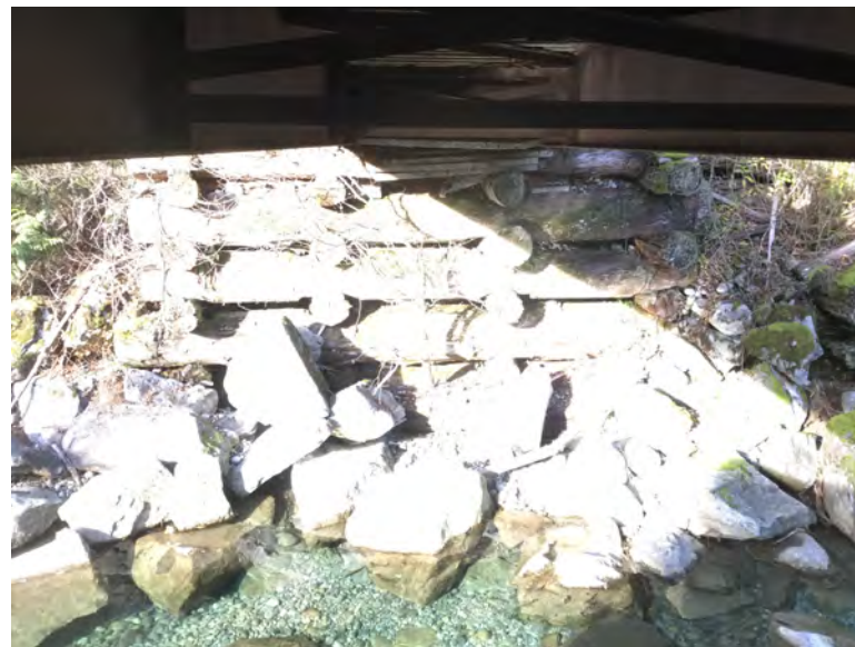
Right Bank Abutment when facing downstream
